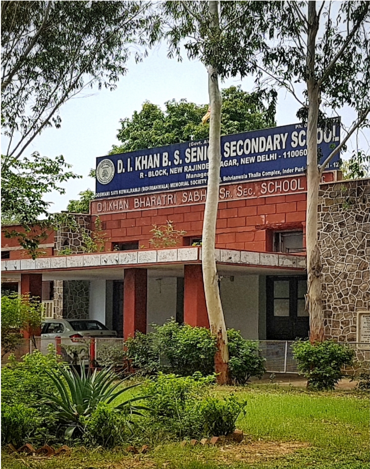
xxxii. Main building of D I Khan Senior Secondary School, located in Rajinder Nagar, Delhi
