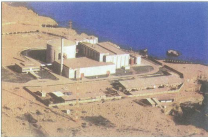
Fig.16.3: Karachi Nuclear Power Plant
