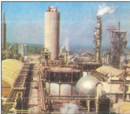
Fig. 12.10: The National Refinery, Karachi
