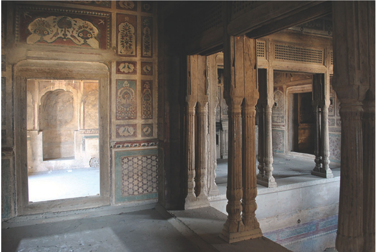
Fig. 12: Wooden columns in the courtyard of Mai Nakain's apartments, Sheikhpura Fort. These pairs of columns are typical of Sikh Empire architecture.
