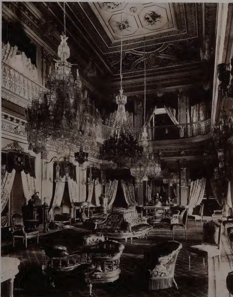
118 Interior of Nizam's Palace, Hyderabad
